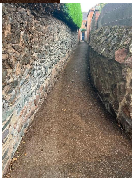
Shooting Close Lane towards Beveridge St
